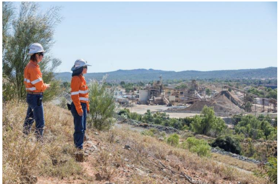
Figure 1 Overview of Processing Plant.
