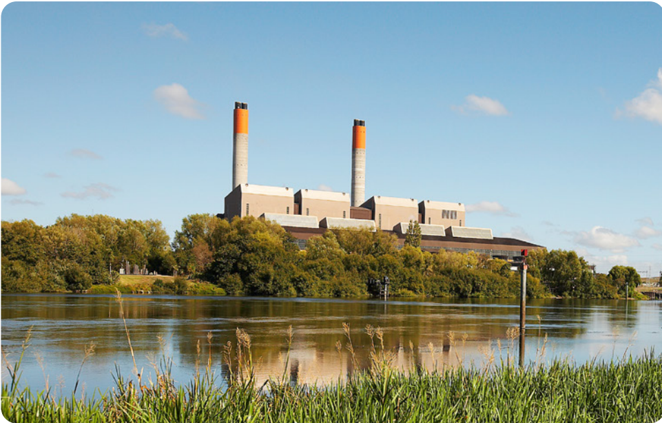
Above: Huntly power station
