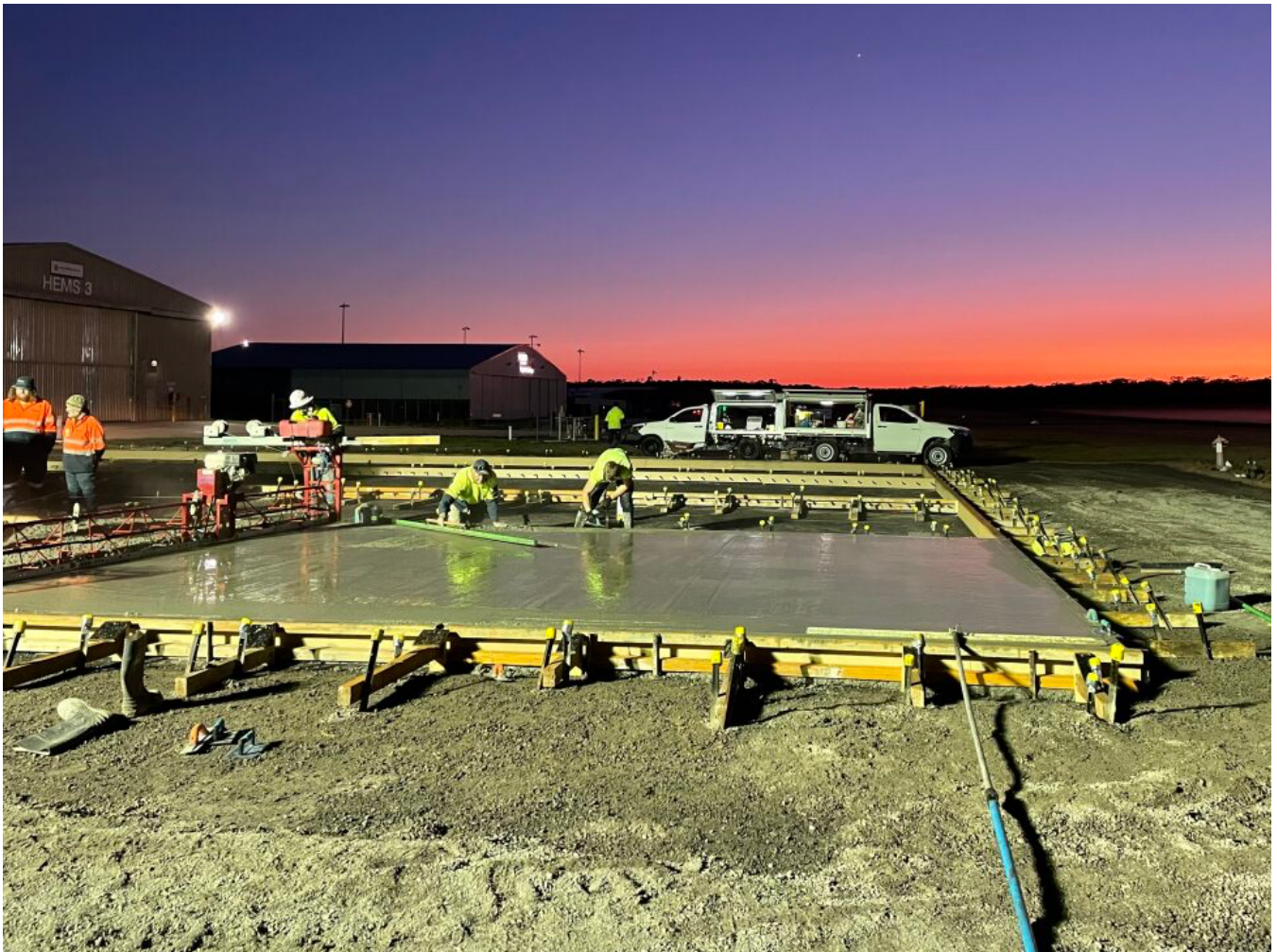
Image: Bendigo Airport Helipad
