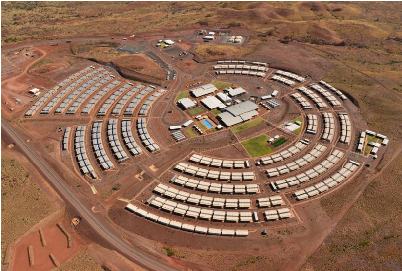
Figure 2 – Roy Hill Mine Permanent Village
