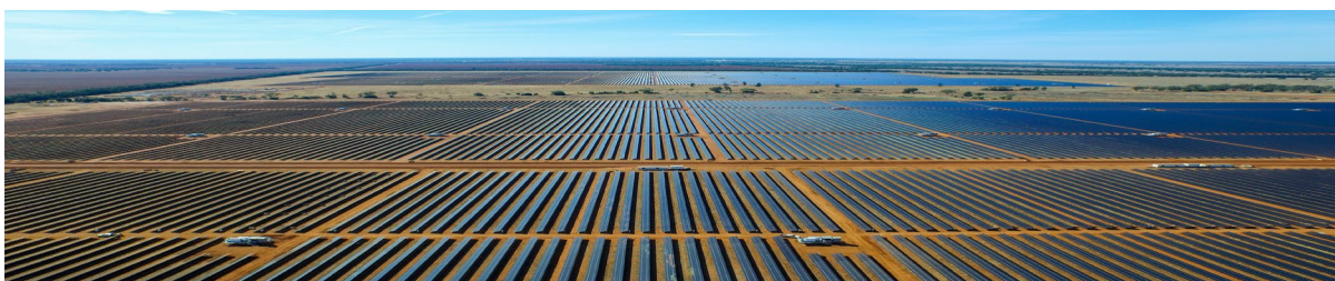
Photo of Nyngan Solar Farm.
