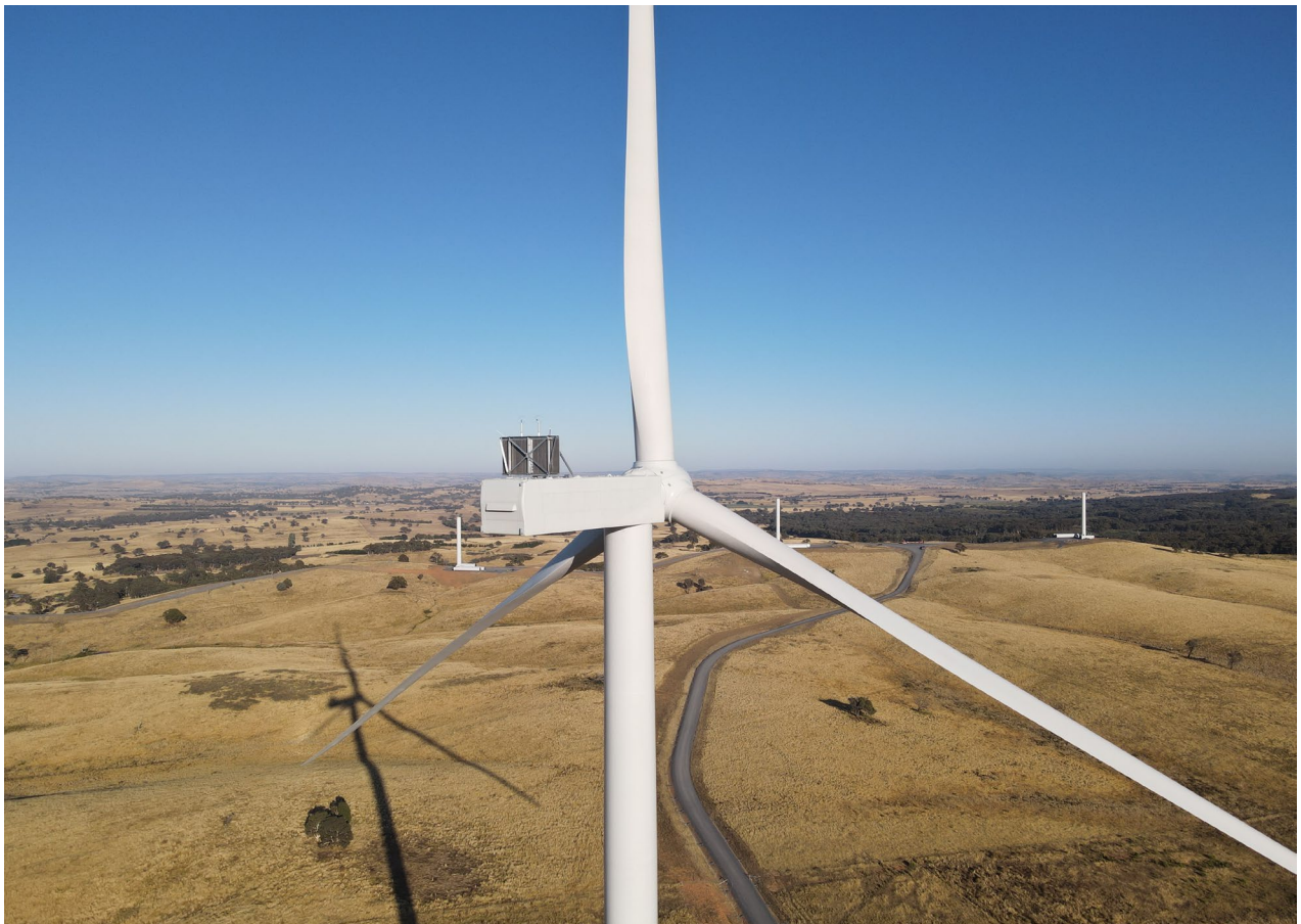
Photo of a Wind Turbine at Dundonnell Wind Farm.
