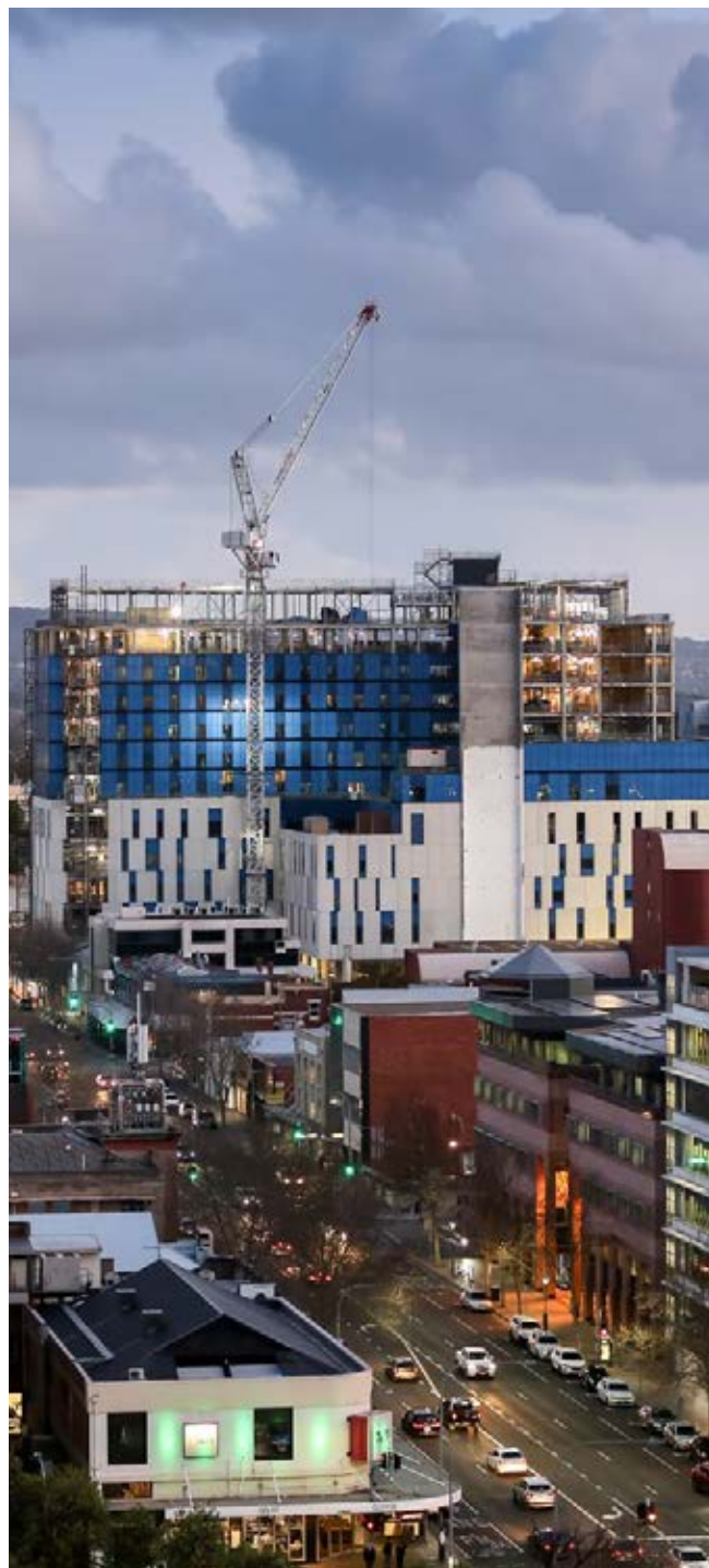
Calvary Adelaide Hospital during construction.
