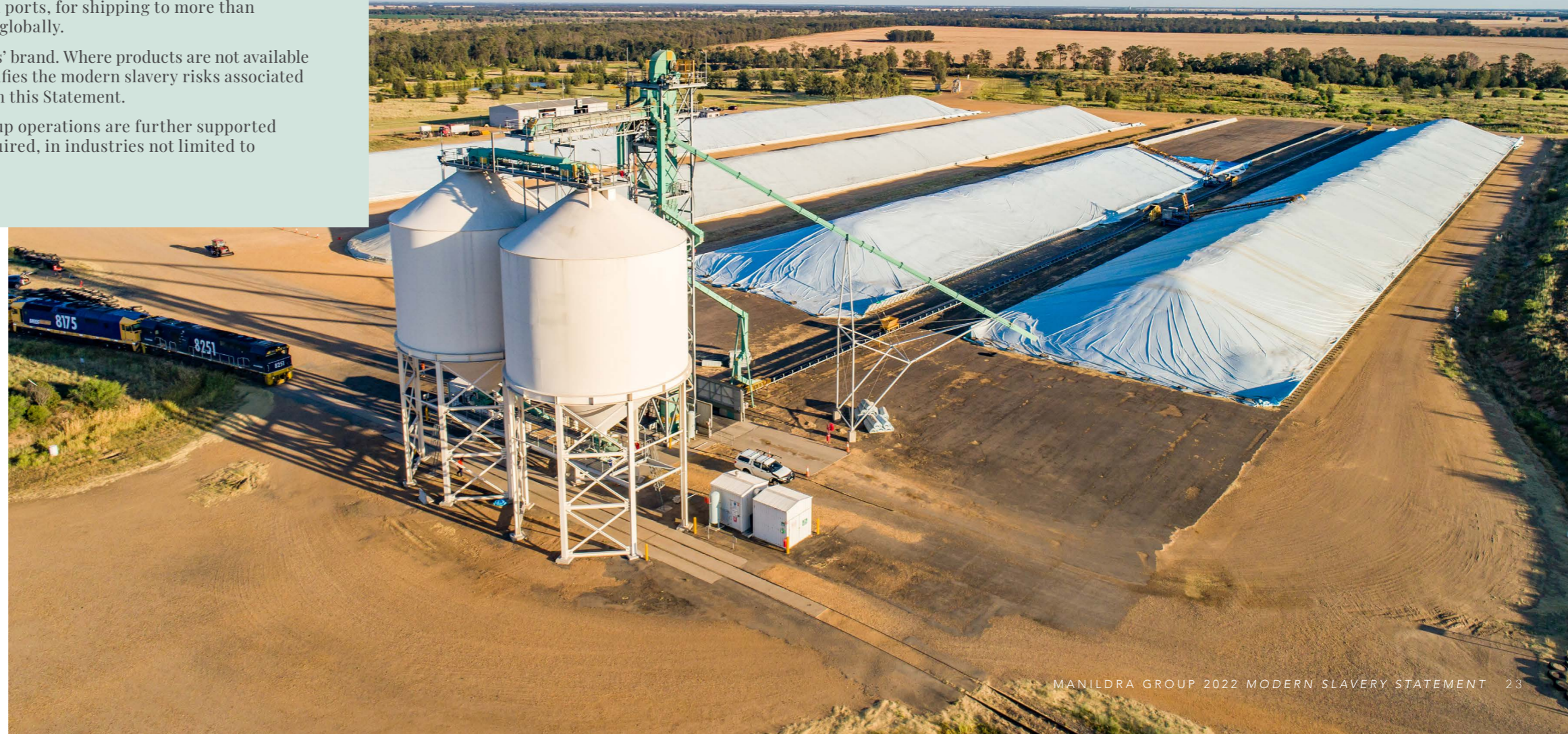
Manildra Group's grain storage site at Bellata, among six grain storage sites we own and operate across New South Wales // PHOTO: CHRIS WATSON
