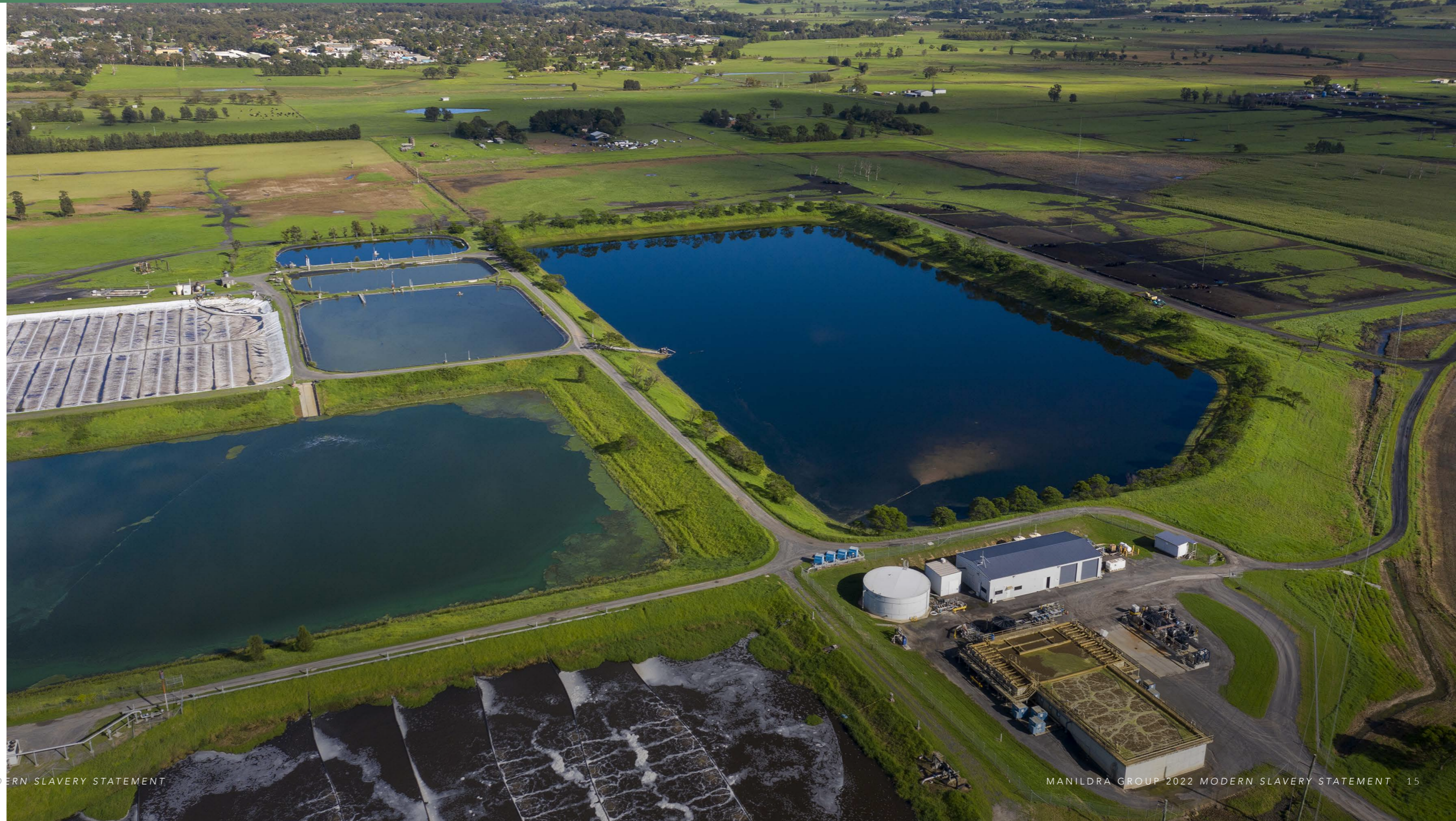
Shoalhaven Starches' integrated Environmental Farm and Water Treatment Plant in Nowra, New South Wales // PHOTO: PETER IZZARD
