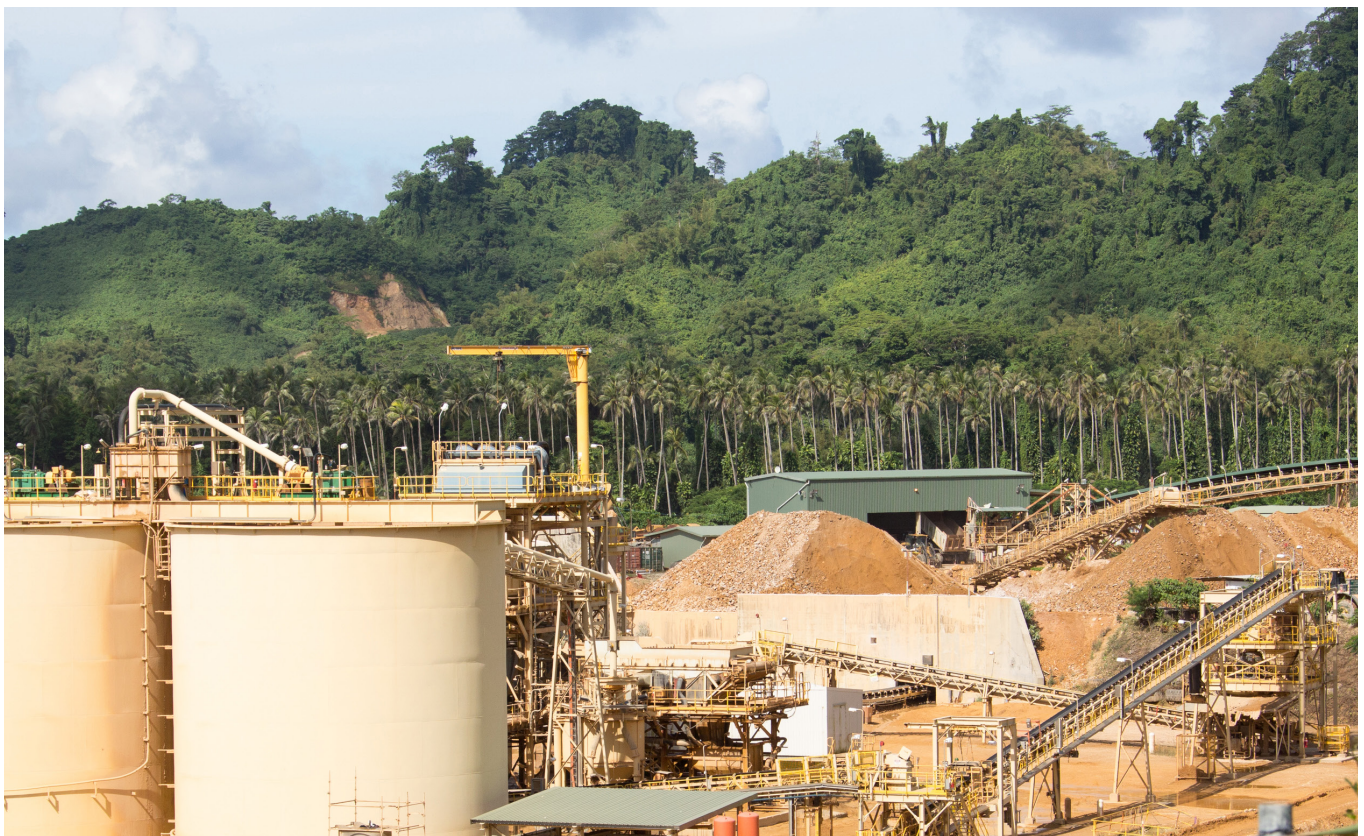
Simberi processing plant
