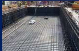
Construction materials (concrete, steel, finishes)
