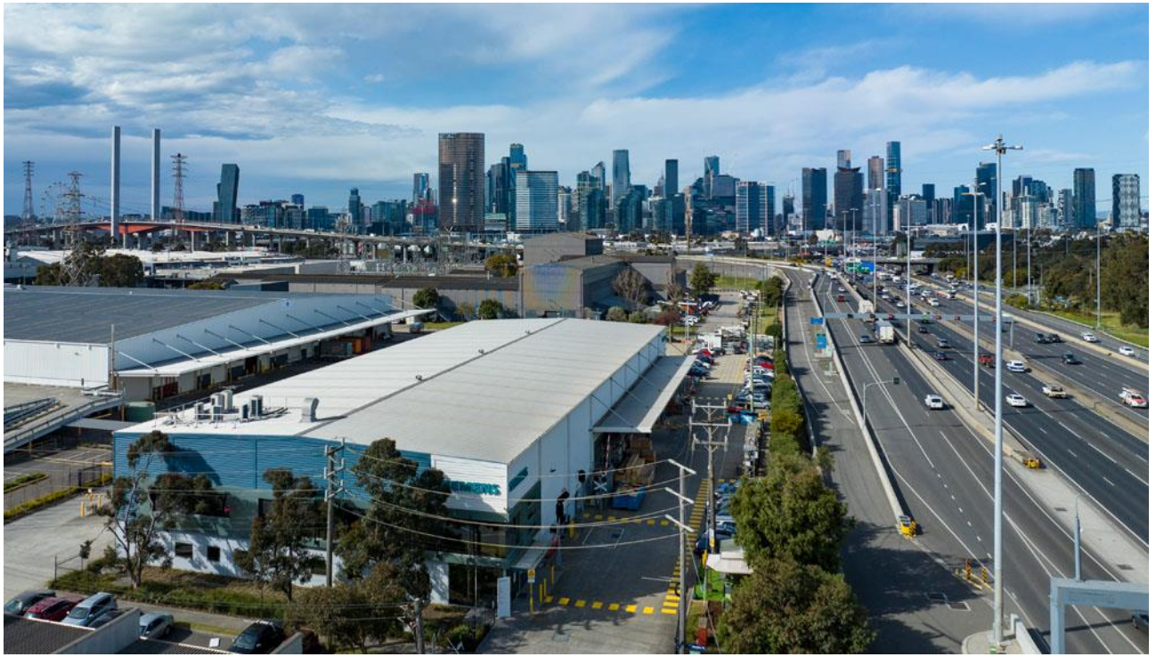
Figure 2 Siemens Mobility Manufacturing Facility in Port Melbourne, Victoria, Australia.
