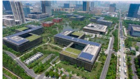
Huawei Hangzhou Research Centre
