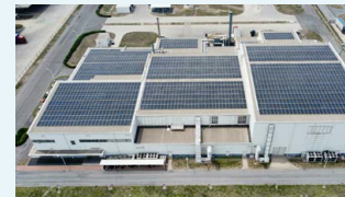
Tianjin packaging factory
