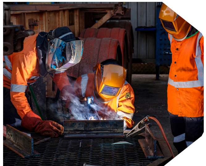
ABOVE: CONSTRUCTION ACTIVITIES ALONG PANAUST LIMITED'S CONCENTRATE HAULAGE ROUTE, LAOS
