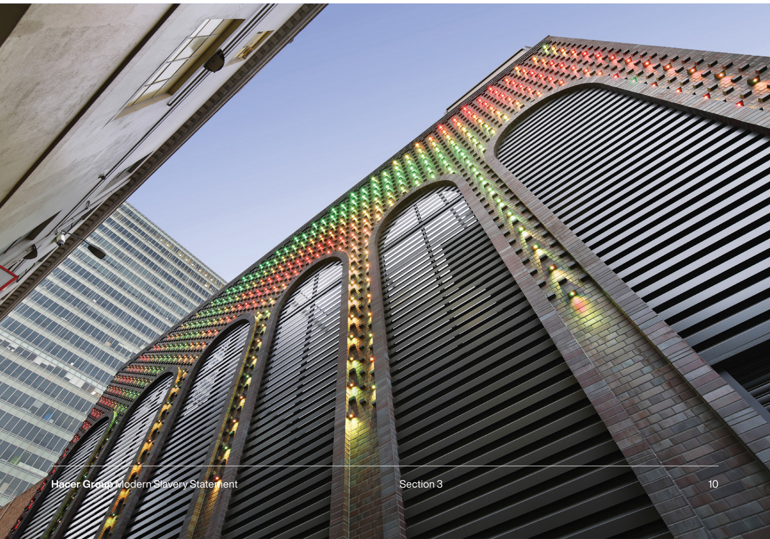
Image: Waratah Place Zone Substation
