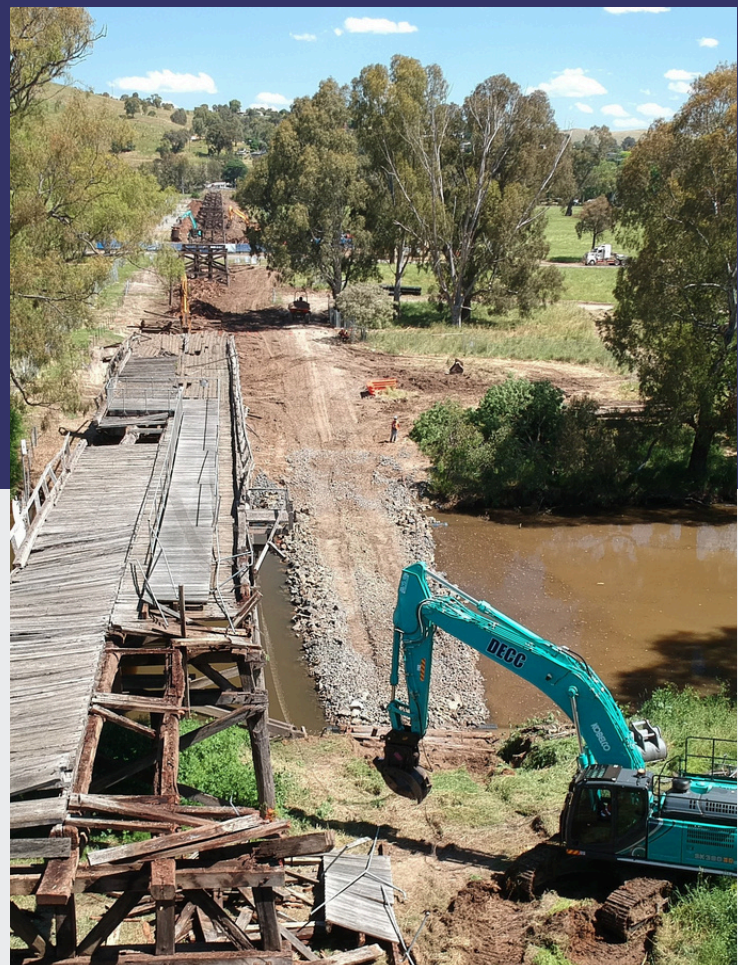
Prince Alfred Via Duct, Gundagai NSW
